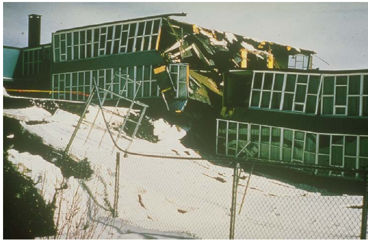
Government Hill Elementary School after the 1964 Earthquake (National Geophysical Data Center)
